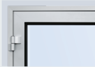
Viewed from inside with synthetic glazing
