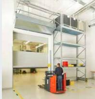
Hörmann high-speed doors are used both inside and as exterior doors to optimise the flow of traffic, improve the room climate and to save energy.
